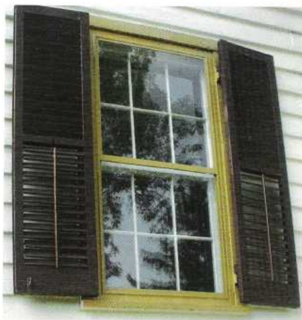
Figure 6. A restored double-hung's authentic divided lights and period glass are visible even behind a storm window. With occasional maintenance, this unit should serve faithfully for another century.
