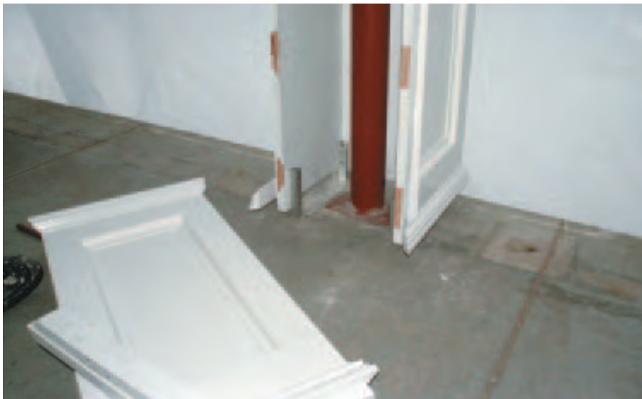
Figure 4. With the jacks and cedar column in position, the three-sided pedestal was slipped into place and fastened with shop-made aluminum hardware designed to stabilize the column while raising it off the floor to prevent moisture problems (above). After the fourth side was biscuited and screwed on, the base moldings were nailed off (right).
