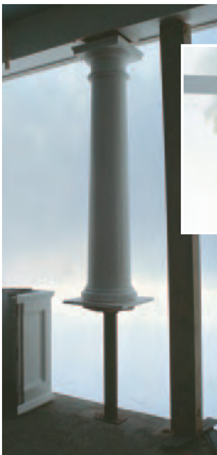
Figure 3. The first step in installing the columns was to slip the cedar column and the top of the pedestal over the screw jack post and position the jack (left). The cedar column was held in place with a clamp-on standpipe bracket, reinforced with a piece of marine plywood (above).
