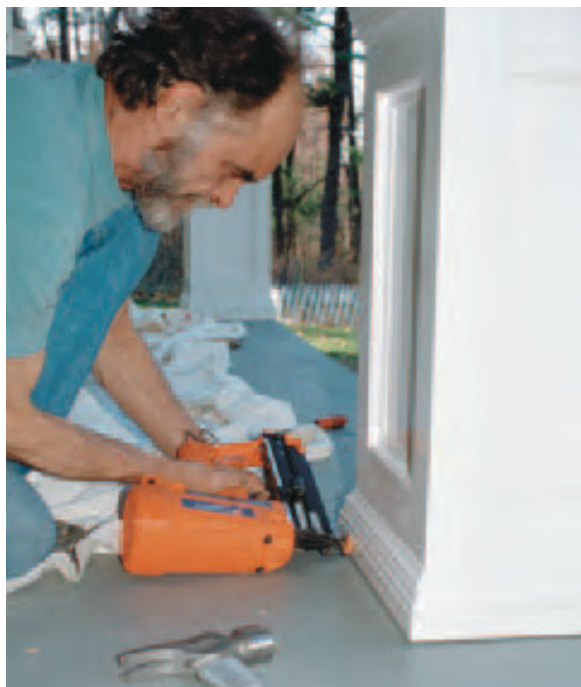
Figure 4. With the jacks and cedar column in position, the three-sided pedestal was slipped into place and fastened with shop-made aluminum hardware designed to stabilize the column while raising it off the floor to prevent moisture problems (above). After the fourth side was biscuited and screwed on, the base moldings were nailed off (right).
