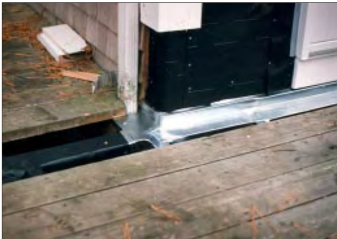
Figure 1. Doubled framing members (top) are good candidates for rot because water that seeps between them cannot drain. In a typical deck repair, the author covers the new double joist with bituminous eaves flashing membrane to keep the water out (above).
