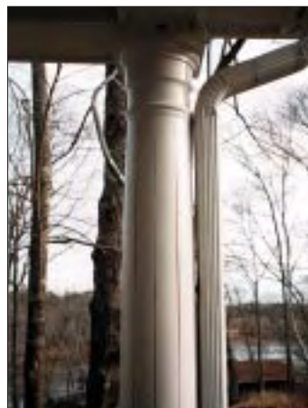
Figure 4. Because wood columns often delaminate (above), the author prefers to use fiberglass columns. They're strong, durable, and easier to install (left).
